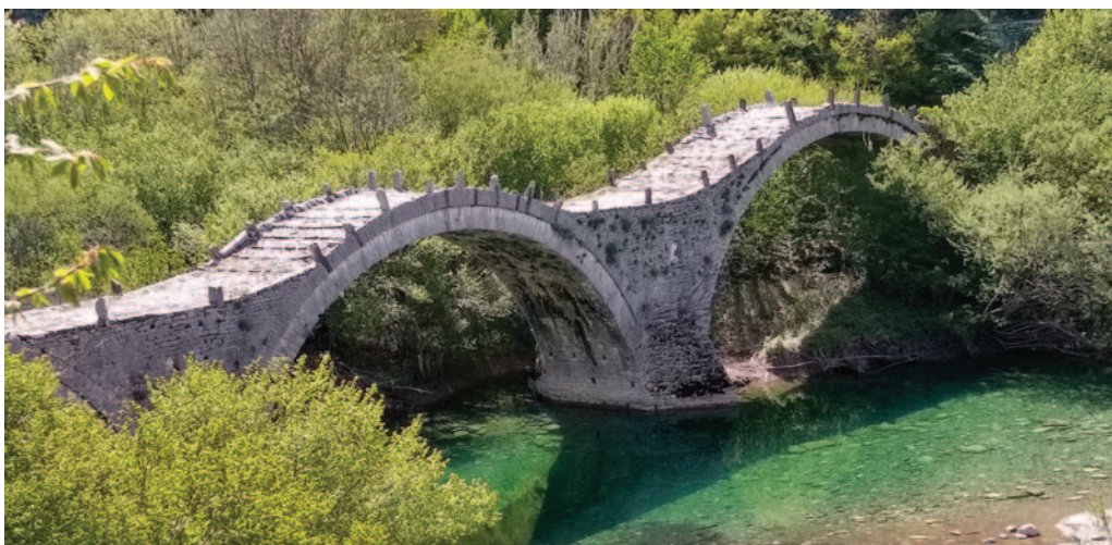
Triple-arched stone bridge dating from the 18th-century in the Zagori region
