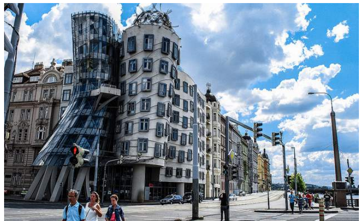
Prague is full of treasures for you to explore in your spare time... this is the "Dancing House" designed by star architects Vlado Milunic and Frank Gehry.
