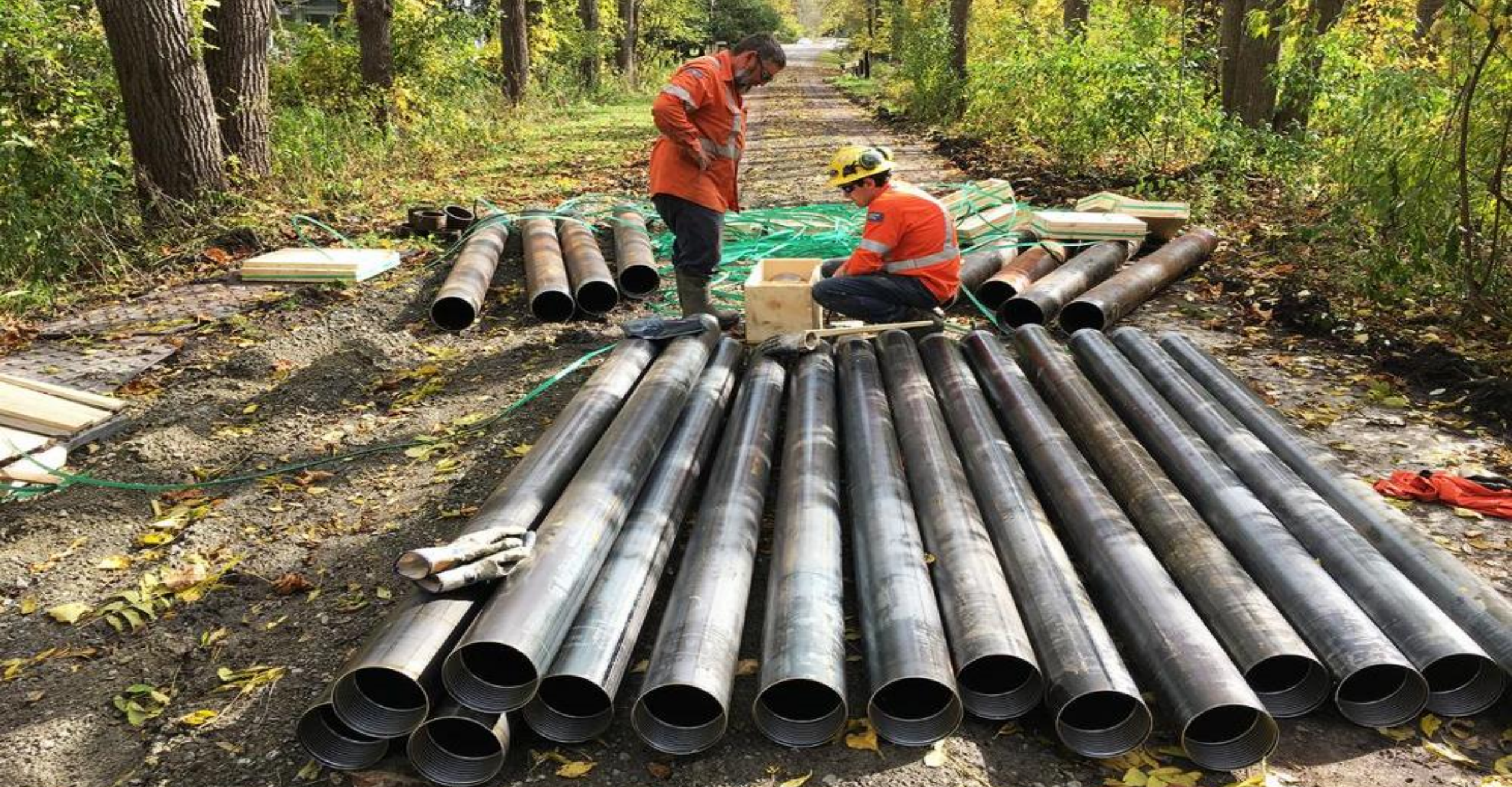
Pipe is drilled down many meters into sediment
