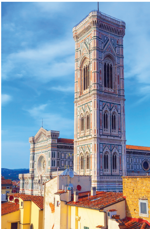
Giotto’s Bell Tower rises above the rooftops of Florence.
